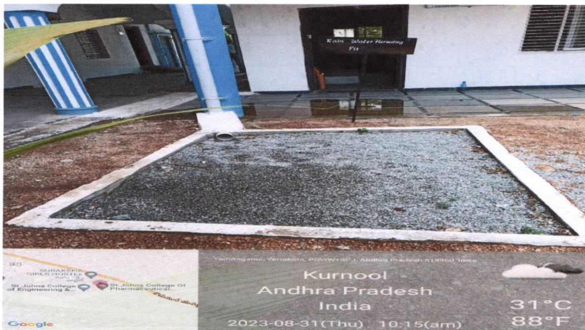
RAIN WATER HARVESTING PIT PHOTO
